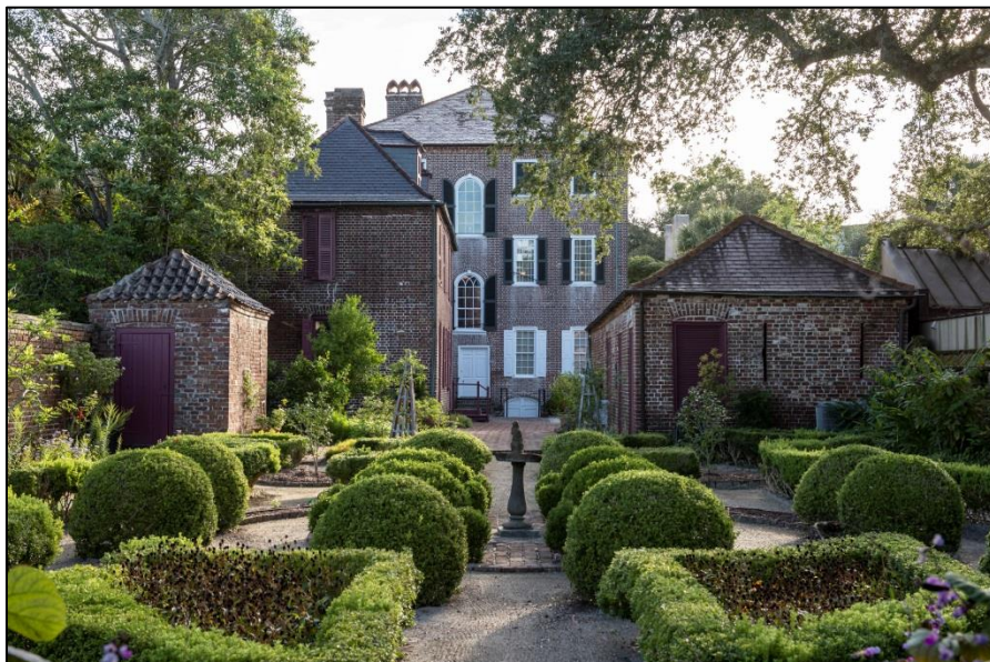
Figure 1-3: Rear view of the Heyward-Washington House, showing the garden, kitchen, stable, privy, and work yard. Collections of The Charleston Museum.
